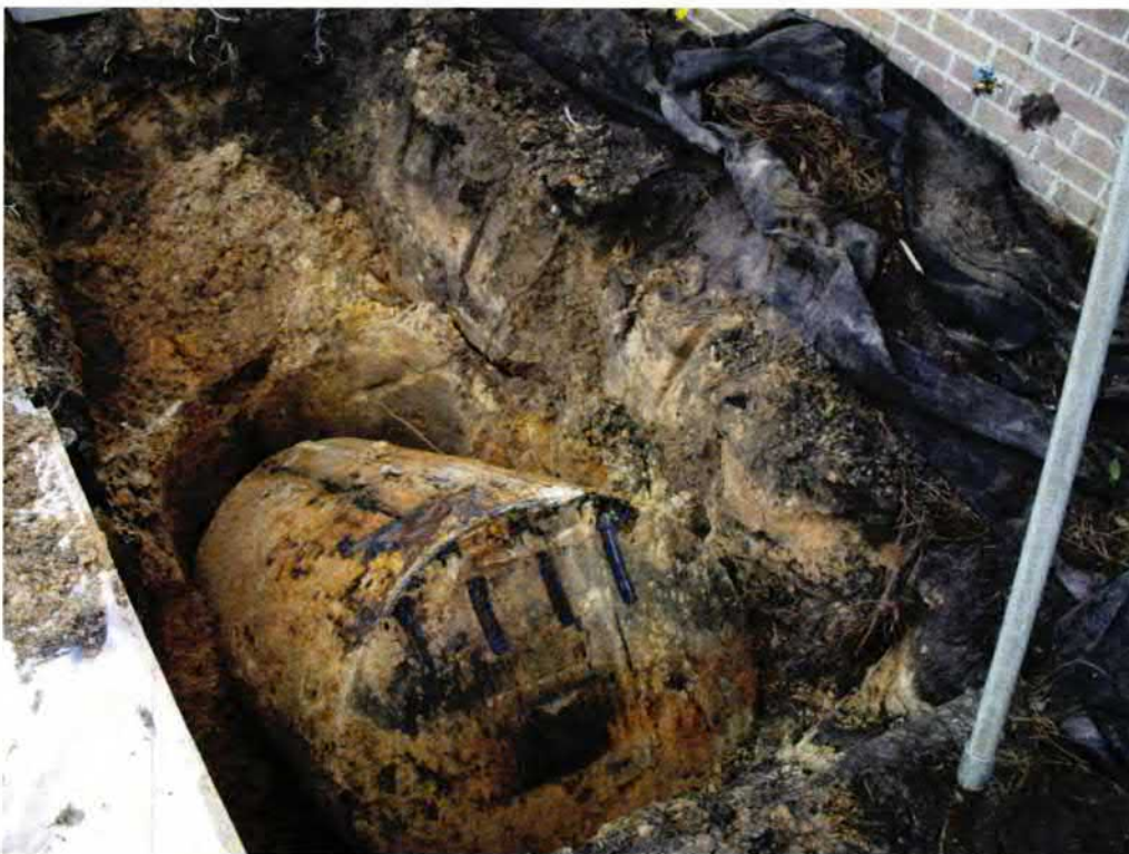
Picture 2: UST 1275 Flamingo excavation during removal.
